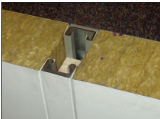
Figure 17: Insulated core panels – internal
